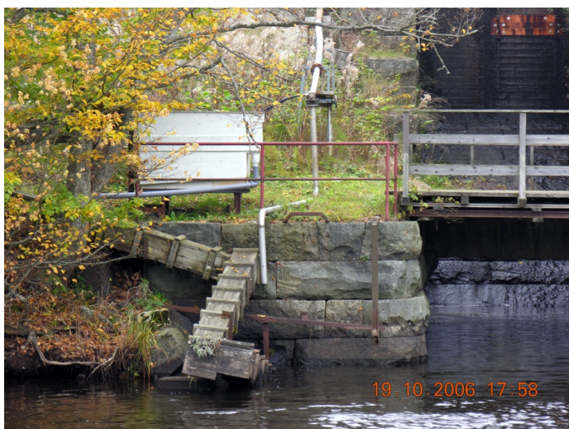
Figure 1 - Eel ladder and collecting box in the River Mörrumsån. The hydropower station is to the right; immigrating eels climb through the wooden boxes filled with wetted substrate (wetted by pipes), ending in the polyester container on top, from which the eels are collected, weighted and then transported upstream.
