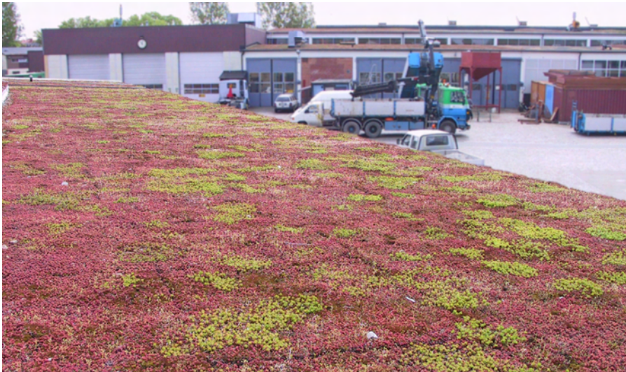
Figure 1. View of a typical extensive vegetated roofs established with vegetation mats. The roof is located on the Augustenborg Botanical Roofgarden
