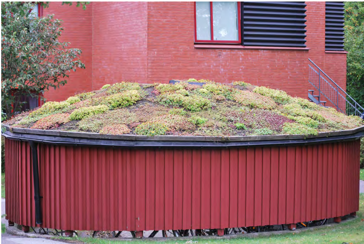
Figure 1 Green roof with sedum blanket
