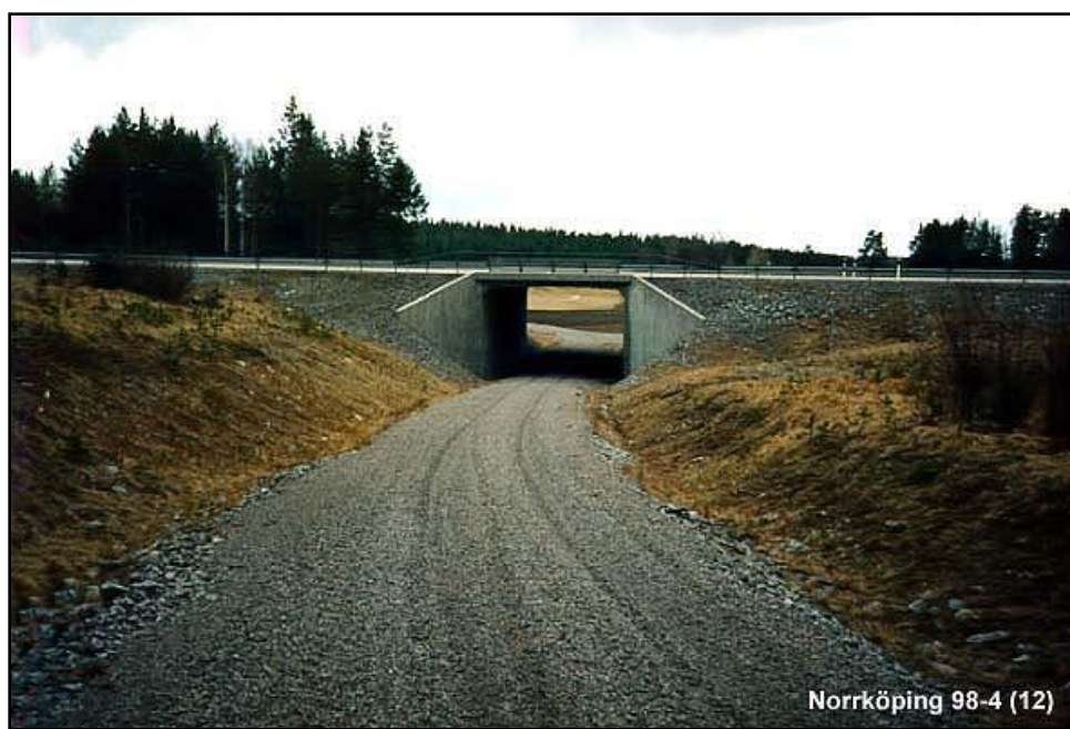
Figure 3: Picture of a typical road underpass for local but publicly used gravel road in Sweden. The picture shows underpass E4N-12 (width 8m, height 5m, length 26m, openness 1.54) that has been completely avoided by moose ( U=0 ), but used to some degree by roe deer ( U=0.32 ), more often by foxes ( U=0.63 ) and very frequently by hares ( U=0.96 ). Photo Andreas Seiler.
