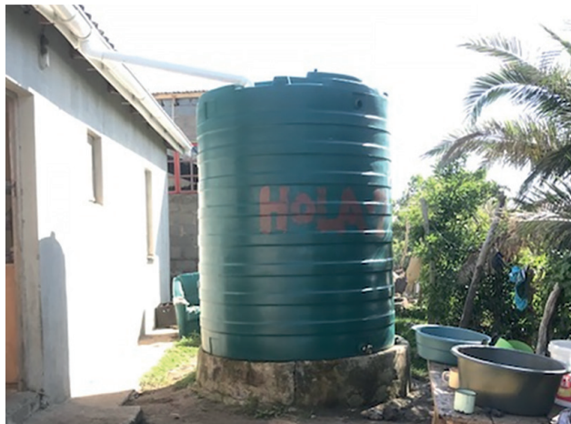
Photo 7: Rainwater tank in Manteku, attached to a downpipe from the tin roof.
