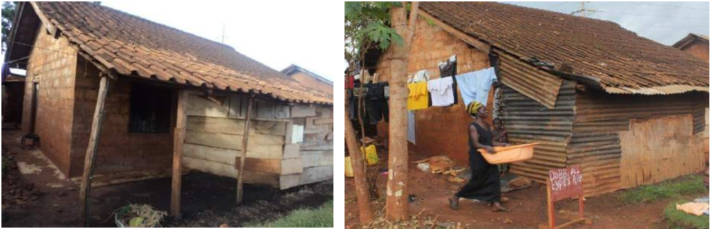
Figure 14. A shed used for charcoal-selling and gradually turned into rented rooms
