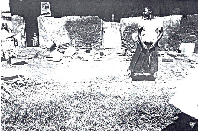
Figure 29. Houses in the study area before the inception of MWSUHP. Source: Wekiya, 1995.
