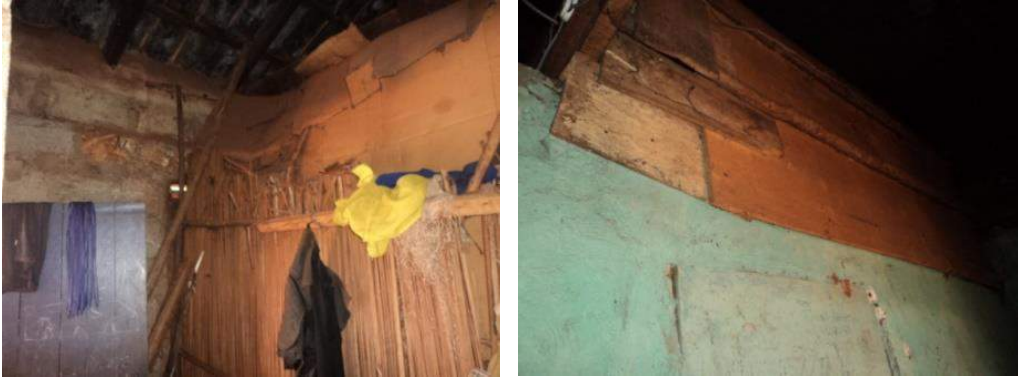
Figure 16. Use of substandard inefficient separating building material compromising privacy and security
