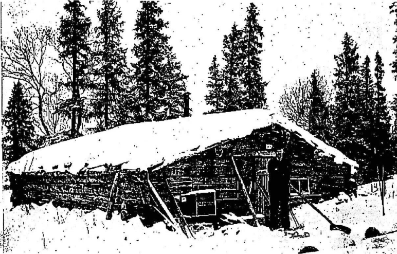
Figure 6. Condemned forestry cabin 1940 (photo: Welin).
