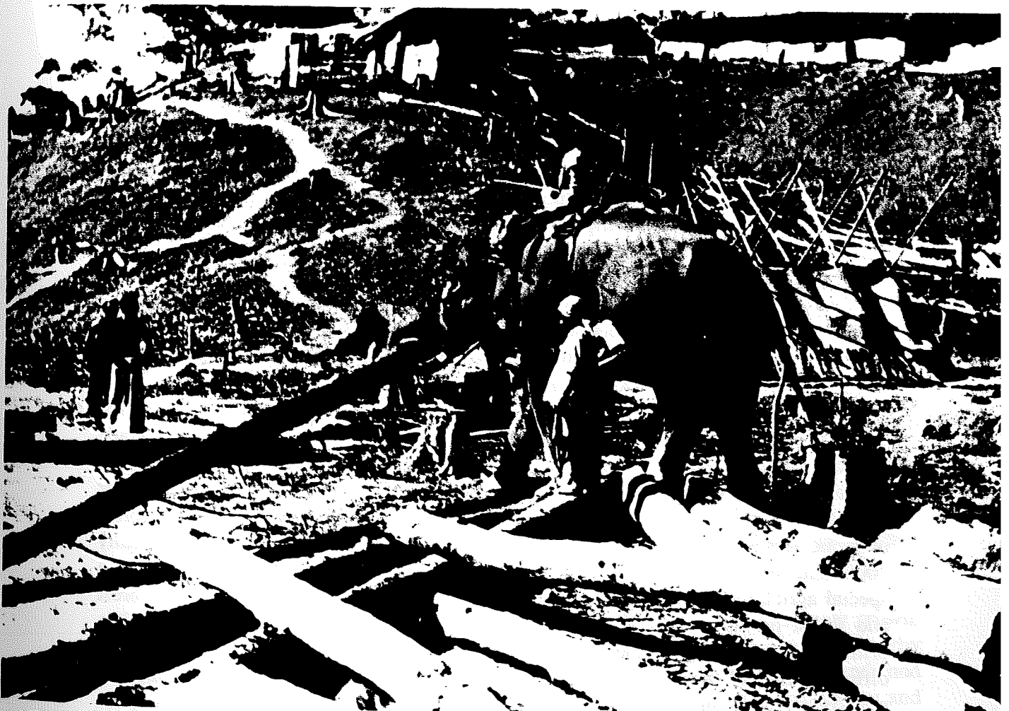
Elephant assembling plantation—grown teak logs preparatory to raft construction on the Karnaphuli River in Bangladesh.
