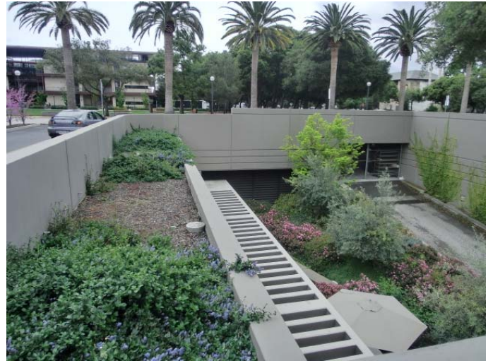
Ventilation behind noise walls
