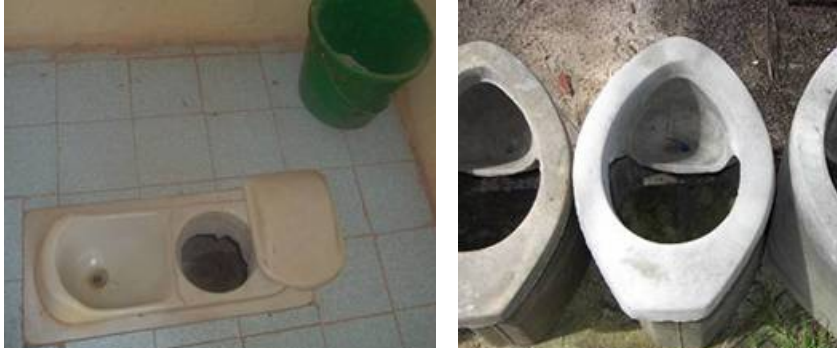
Fig. 3. Dry urine-diverting toilets, Left: Squatting type; Right: Pedestals, Uganda (photos: C. Niwagaba, 2004).
