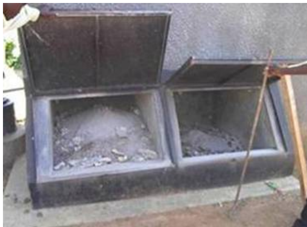
Fig. 5. The faecal collection chamber of a dry urine-diverting toilet showing the heap formed by the faeces, cover material and wiping material (photo: C. Niwagaba, 2004).
