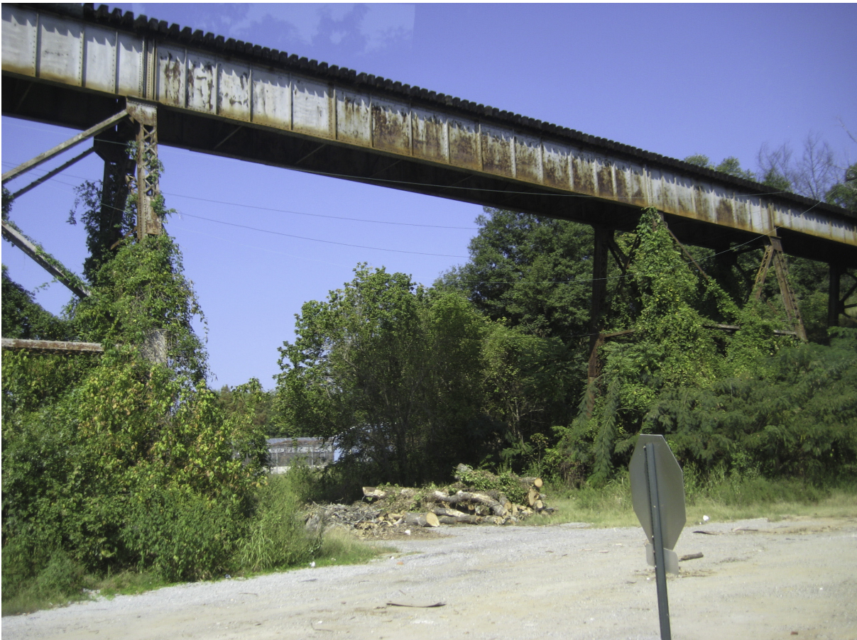
Fig. 2. Abandoned railroad bridge
