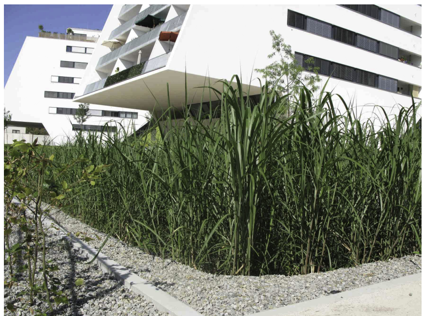
Fig. 2 Inconspicuous open storm water drainage – Bombadier estate in Vienna, Austria, by Rajek Barosch Landscape Architects
