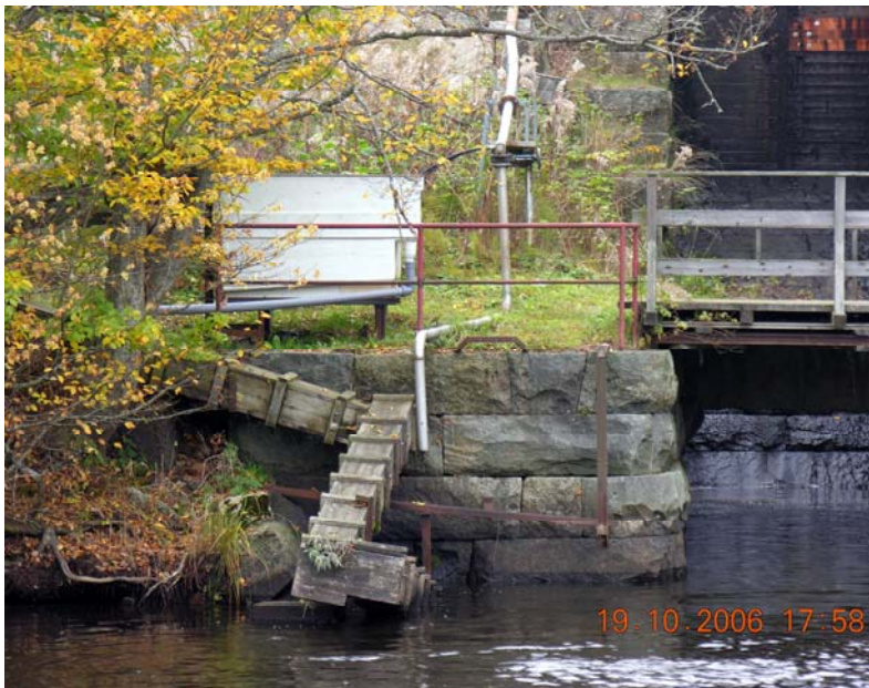
Figure 5 - Eel ladder and collecting box in the River Mörrumsån. The hydropower station is to the right; immigrating eels climb through the wooden boxes filled with wetted substrate (wetted by pipes), ending in the polyester container on top, from which the eels are collected, weighted and then transported upstream.
