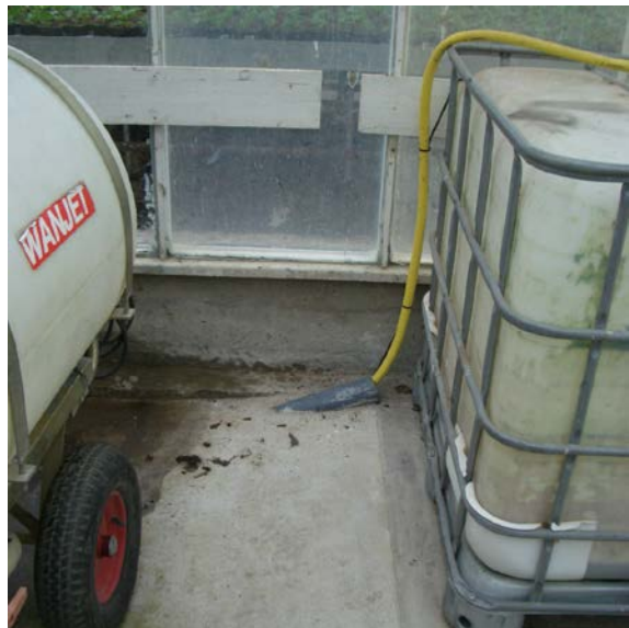
Fig. 8. Working place with a sump pump pit, connected to a separate waste tank.
