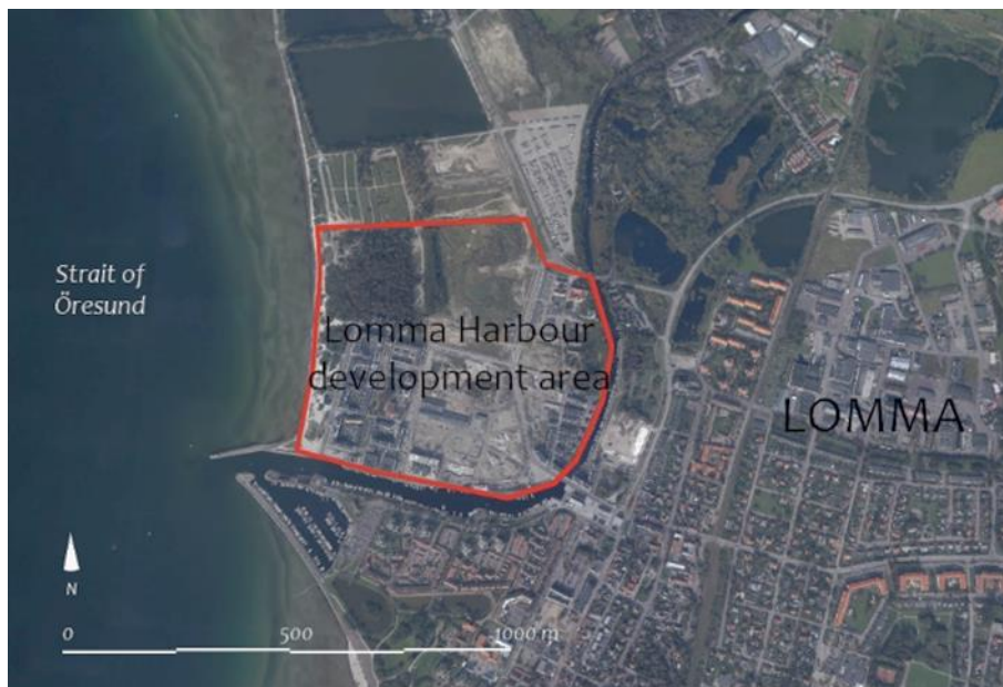
Figure 6. Aerial photograph of the Lomma Harbour development area in Lomma, Sweden.
