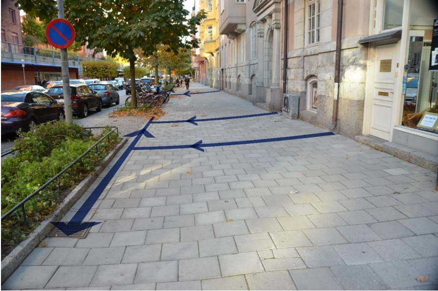
Figure 4. An examples of SuDS where surface runoff is connected to the planting beds and the runoff is used as a resource to water the trees (Stockholm, Sweden) (Sjöman & Slagstedt, 2015).
