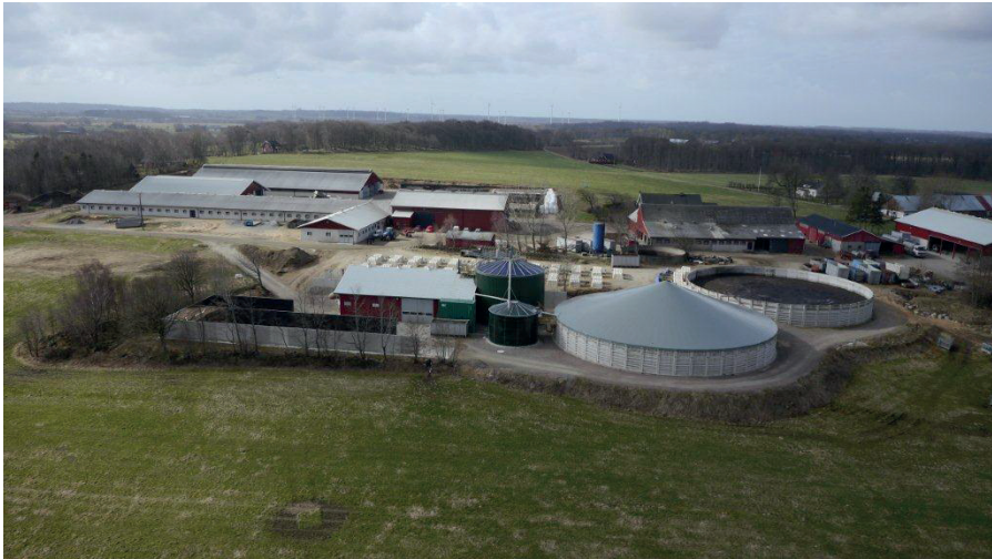
Figure 5. Aerial view of a Swedish farm-scale biogas plant (FSBP) with, main digester, second digester, covered storage and final uncovered storage. Photo: Mattias Bergström.
