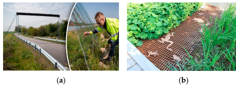
Figure 4. (a) A new road (serving an urbanized countryside) destroys the domain of the protected hazel mouse. To mitigate the effect, the traffic board installed a bridge for the mice to use. Two years after installation, the vegetation is not sufficient to make the bridge work as intended. (Photo: Skåne County Council website, visited 2019-05-30). All rights reserved) (b) To keep the rules for biodiversity in the National City Park in Stockholm, when building an adjacent dense urban district, a frog tunnel must be constructed, to allow frogs to move freely under streets and between and inside raingardens and ditches. (Photo: SWECO website, visited 2019-05-30).
