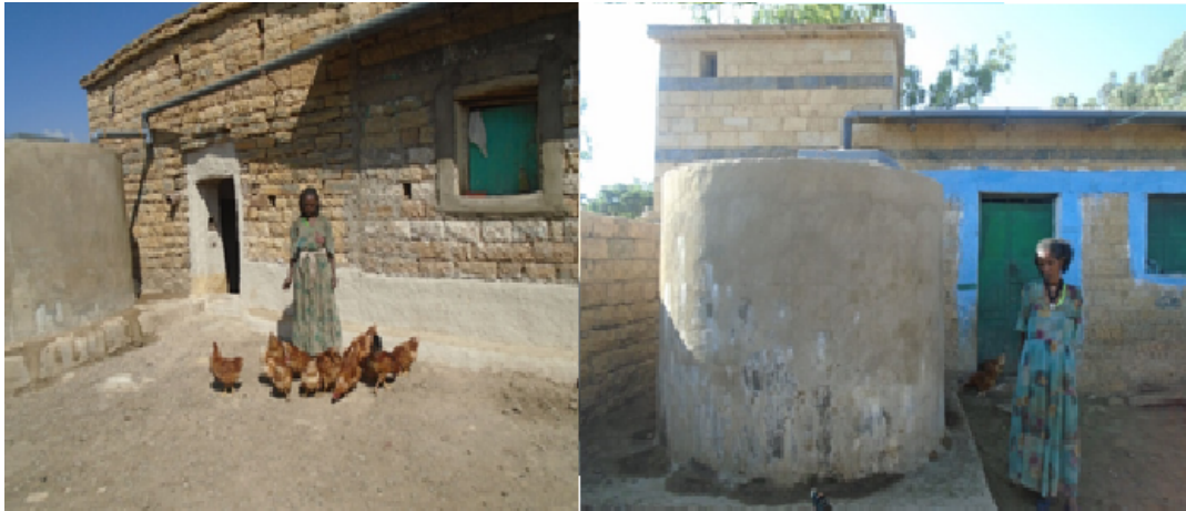
Figure 4. Household roof water harvesting (source: Mulu Haftu)
