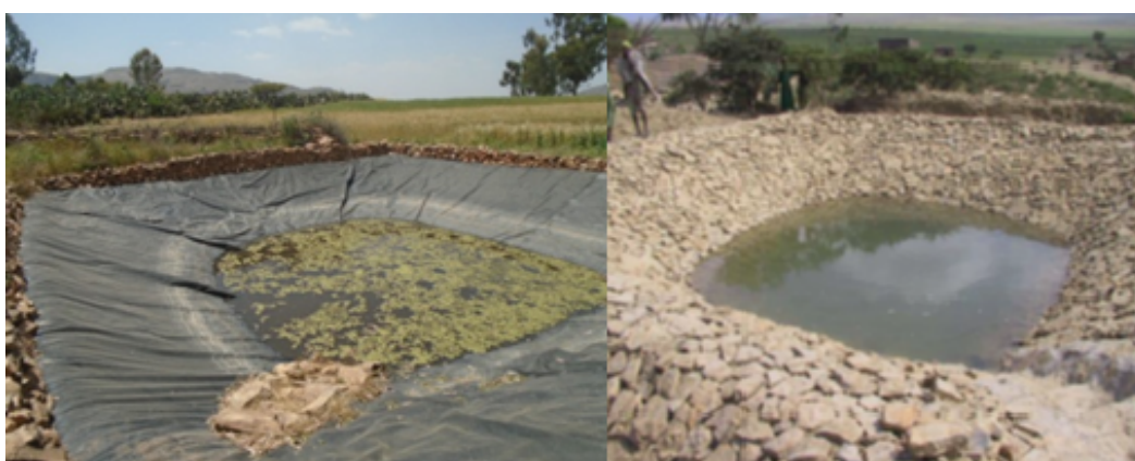
Figure 2. Household pond 'horeyo', black polyethylene membrane lined (left) and cement plastered/rip rap (source: Mulu Haftu)
