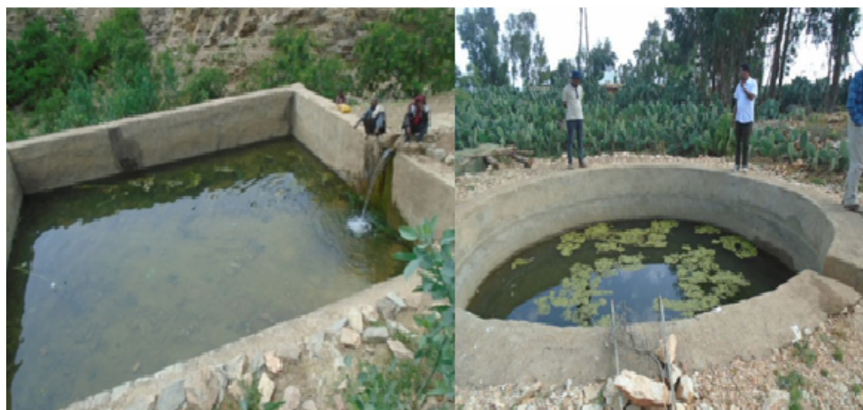
Figure 3. Household Tanker (rectangular and hemispherical tanks) (source: Mulu Haftu)
