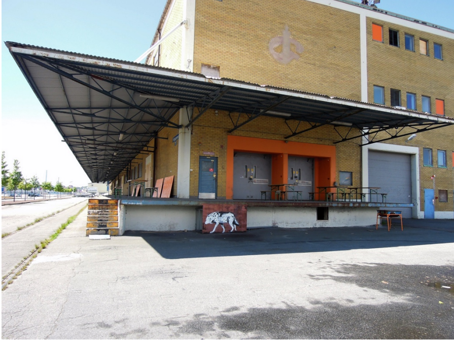
Figure 18. Cantilevering structures used as a prototype for events at Frihamnen in Gothenburg, Sweden. (Photo: Caroline Dahl)
