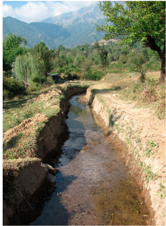
Figure 5. The canal was desilted and widened to improve water flow.
