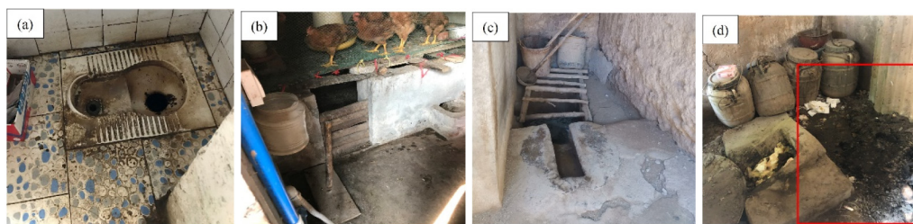
Use interface: a) Stained source separation toilet, b) toilet and livestock in the same space, c) septic-tank and interface in the same room, and d) mixture of soil and excreta placed in the toilet.
