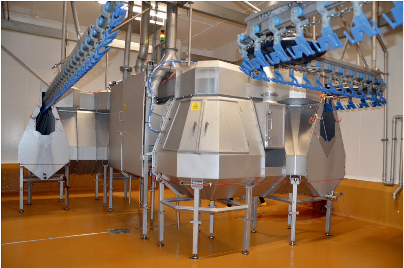
FIGURE 1. Ultrasound-steam chamber installed in the slaughter line of a large-scale broiler chicken processing plant.
