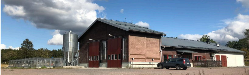
Figure 1. The laying hen facility at Lövsta Research Centre outside Uppsala.
