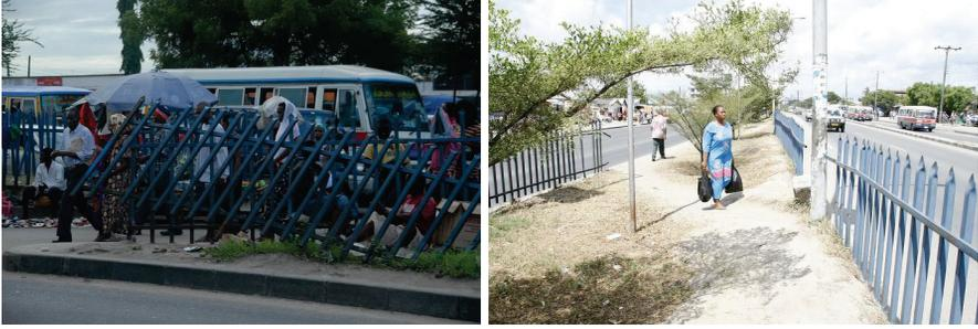
Figure 25. Broken barrier which had been constructed to direct pedestrians to use the overpass bridge along Morogoro Road to avoid accidents and traffic jams.
