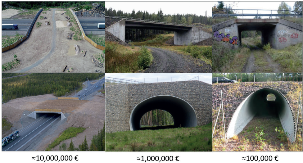
Figure 1. Examples of differently sized crossing structures in Sweden used by large wildlife, with rough estimates of investment costs. The precise costs depend on a number of site-specific factors, and values given are intended to serve as indications. Images by courtesy of Trafikverket and PEAB.
