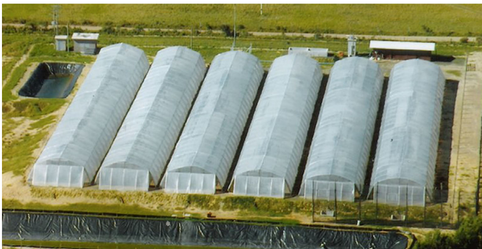
FIGURE 4 Bio-RAS with six greenhouse fattening reactors, recirculation tank (bottom) and denitrifying tank or sludge concentration/reuse tank (top left). Photo: Sergio Zimmermann (2003).
