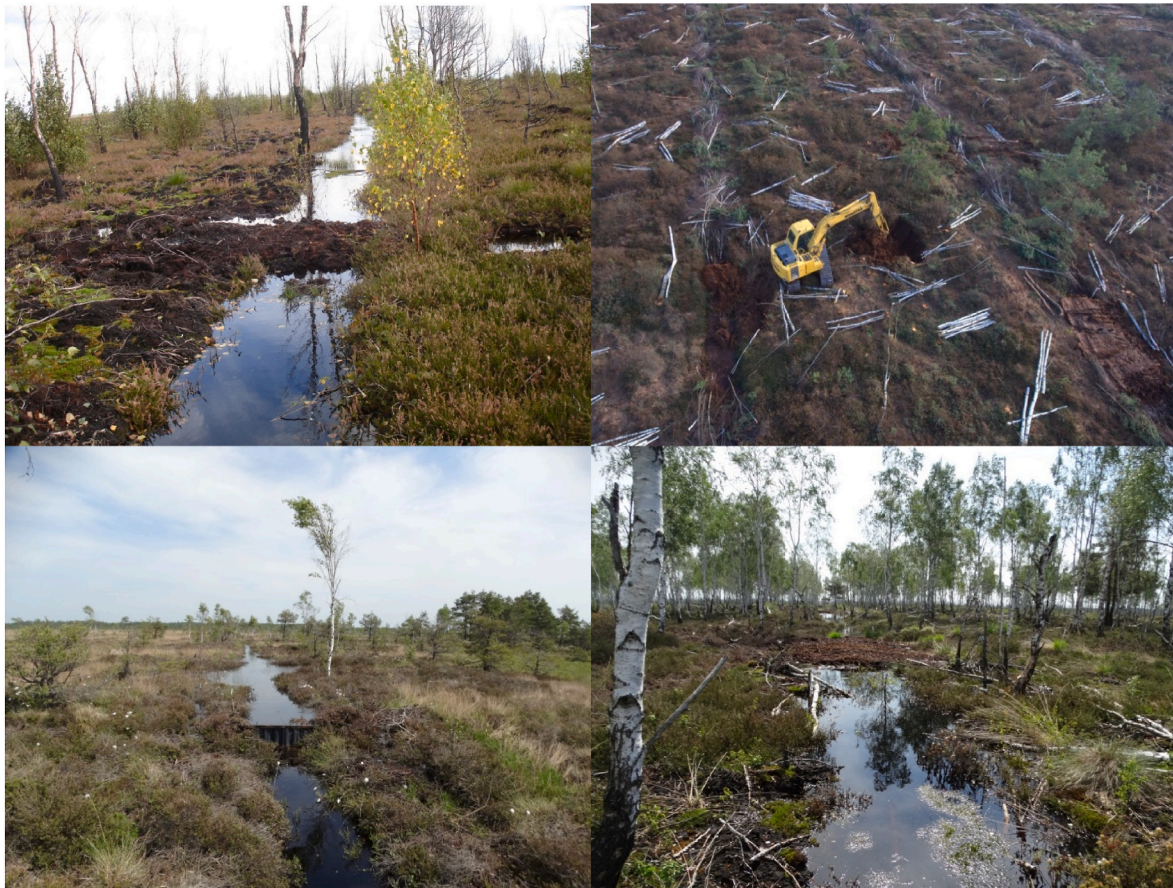
Fig. 3. Peatland rewetting and restoration using ditch blocking to raise the water table and water storage capacity in Aukštumala raised bog, Lithuania, photos by L. Jarašius and J. Sendžikaitė.
