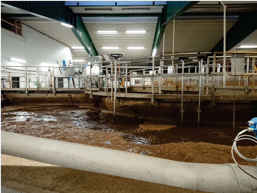
Figure 7 Site photo of the pre-treatment reservoir sampled at the Kivik WWTP. View of the pre-treated wastewater influent to the disc filtration treatment step at the Kivik WWTP (Appx III - Paper III). Photo credit: Maria Yu
