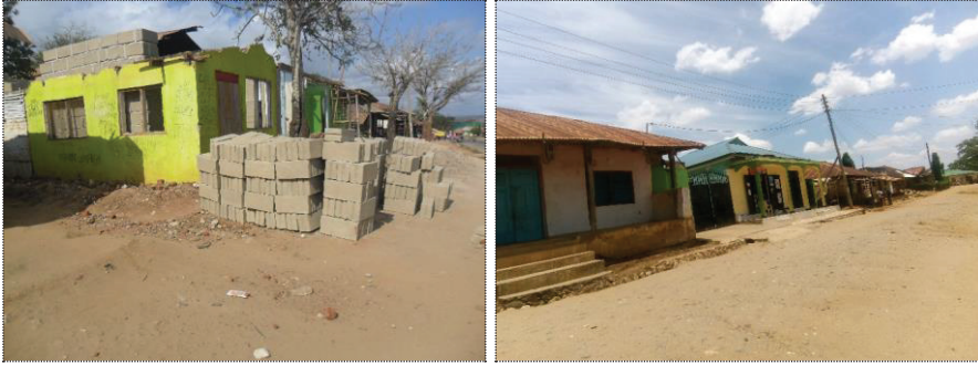
Plate 3. Building reconstruction in Handeni town Source: Fieldwork 2018
