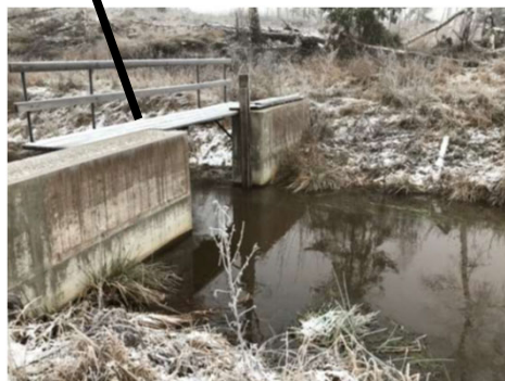
Figure 4. Dam to block the ditch and raise the water table.
