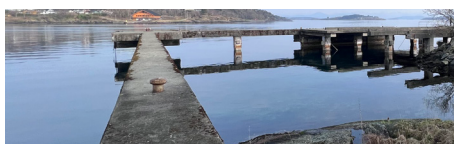
2 and 3. Pier construction at the water edge (from 1950s/60s)
