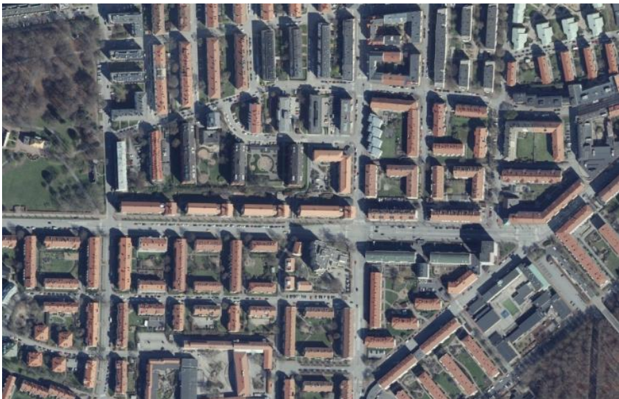
Figure 7. A typical neighbourhood in the urban setting. Aerial photo from Lantmäteriet ©
