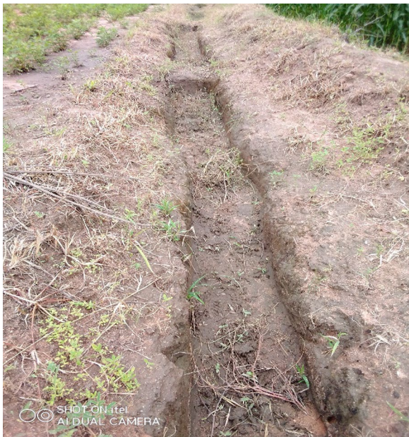
Fig. 5 STDC ridges reinforced with variants of infiltration pits in Marange with dimensions of 5 × 0.5 × 0.5 m for Length x Width x Height. (Photos by George Nyamadzawo)
