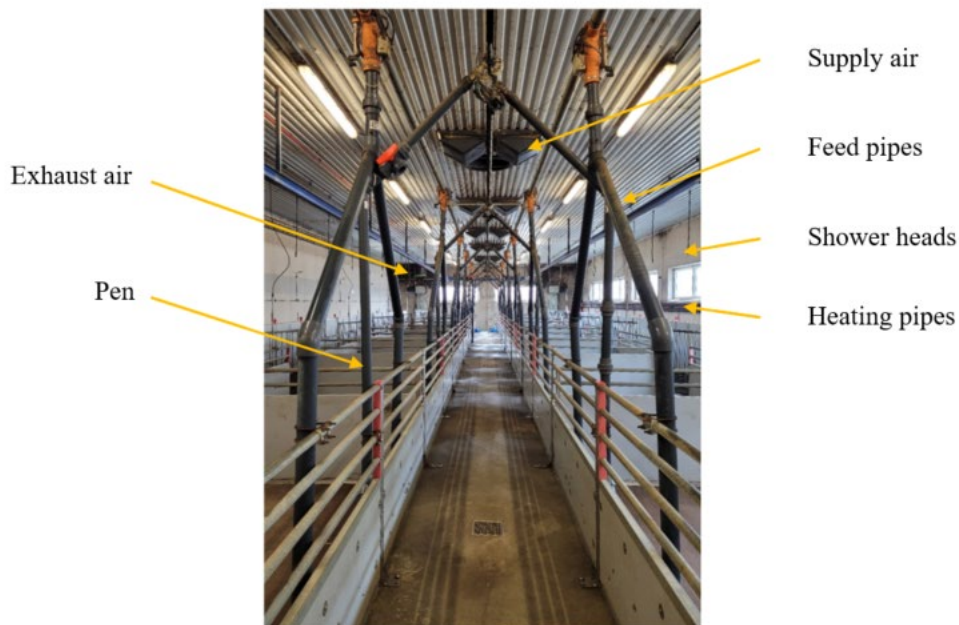
Figure 5: Typical layout in a Swedish livestock building for pigs, including one exhaust fan, one ceiling air jet per pen, pipes for feed, heat pipes below windows, and showers for cooling and dust binding (Farm visits 2022-2023).
