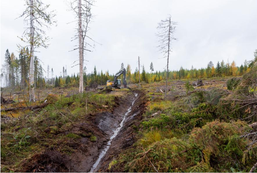
Figure 3. Excavator cleaning a ditch in Trollberget, northern Sweden (photo credit: Andreas Palm).
