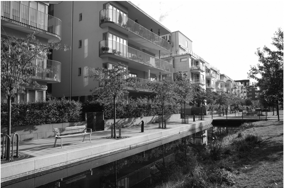
Figure 6. Homes in Hammarby Sjöstad. In the foreground is a channel that is part of the storm water system. The large windows provide an attractive lake view, but are in conflict with the objective to keep energy consumption down. (Photograph: the author, 2008)
