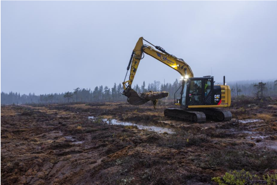
Figure 4. A ditch being filled during the restoration of the Stormyran mire, in the Trollberget study site. Image credits: Andreas Palmén.
