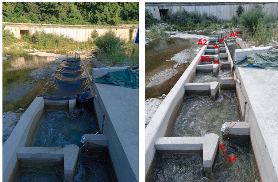
Fig. 2. The vertical slot fishway in covered (left) and open (right) conditions. In the foreground the uppermost antenna (A4) and test tag are visible on both photos. The position of the four antennas (A1–A4) is indicated in red on the right. (For interpretation of the references to colour in this figure legend, the reader is referred to the web version of this article.)
