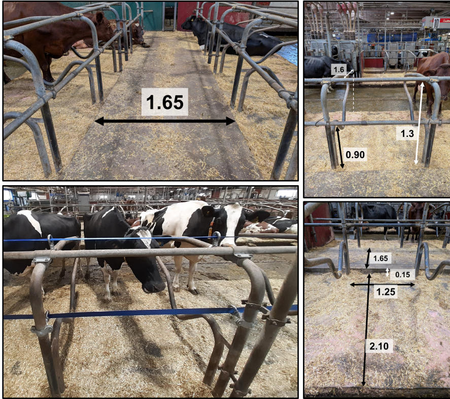
Figure 4. Cubicle design and dimensions (meters). Flexible head and neck straps in the lower left quadrant.
