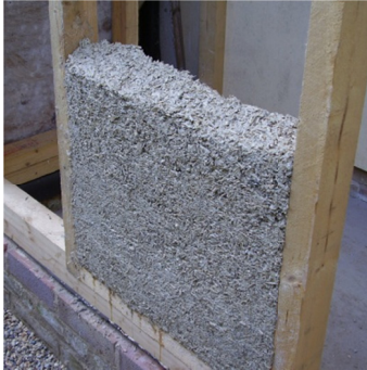
Figure 1. Tamped hemp after the removal of temporary shuttering. (Picture: P.B. de Bruijn).
