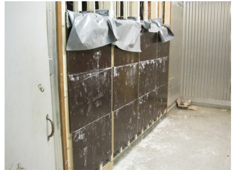
Figure 21. The wall has been built; plastic film was put on top to prevent the wall from drying too quickly.
