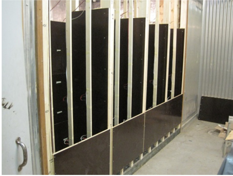
Figure 18. Mould for the wall, ready to be built. Pieces of masking tape indicated how far one batch should reach.
