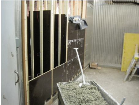
Figure 20. The mould for the wall, half the wall is built. In the foreground a new batch of LHC.
