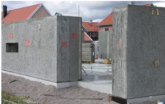
Figure 13. Wood-wool cement wall elements on a building site in Dalby, Sweden. (Picture: M. Rückert)
