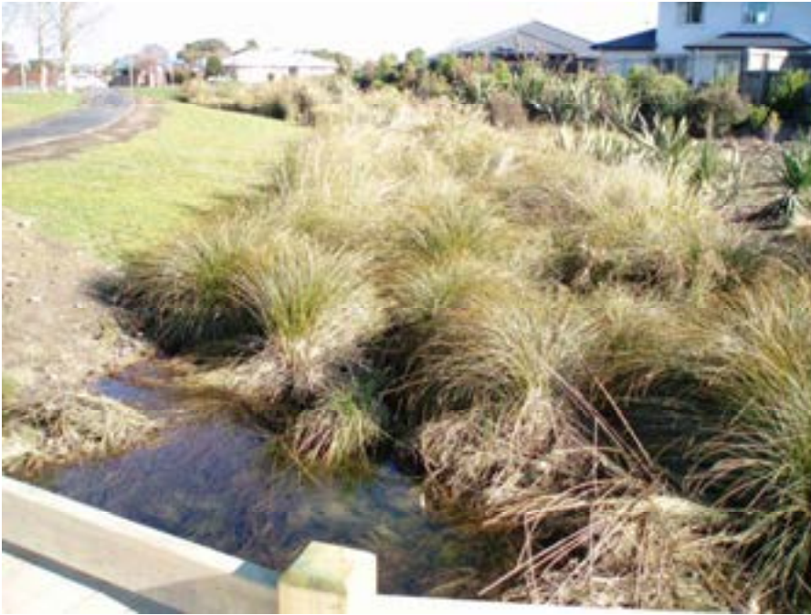
Picture 46. Aidenfield, Christchurch – swale treatment of stormwater in a greenfields, low impact urban development. The swale has been planted with filtering beds of indigenous sedges, rushes and NZ flax, with shrubs and small trees on the shoulders.
