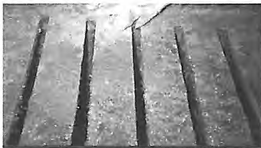
Figur 6. Betongspalt, 25 mm öppning (sinsuggspalt). Figure 6. Slatted concrete floor, opening 25 mm.
