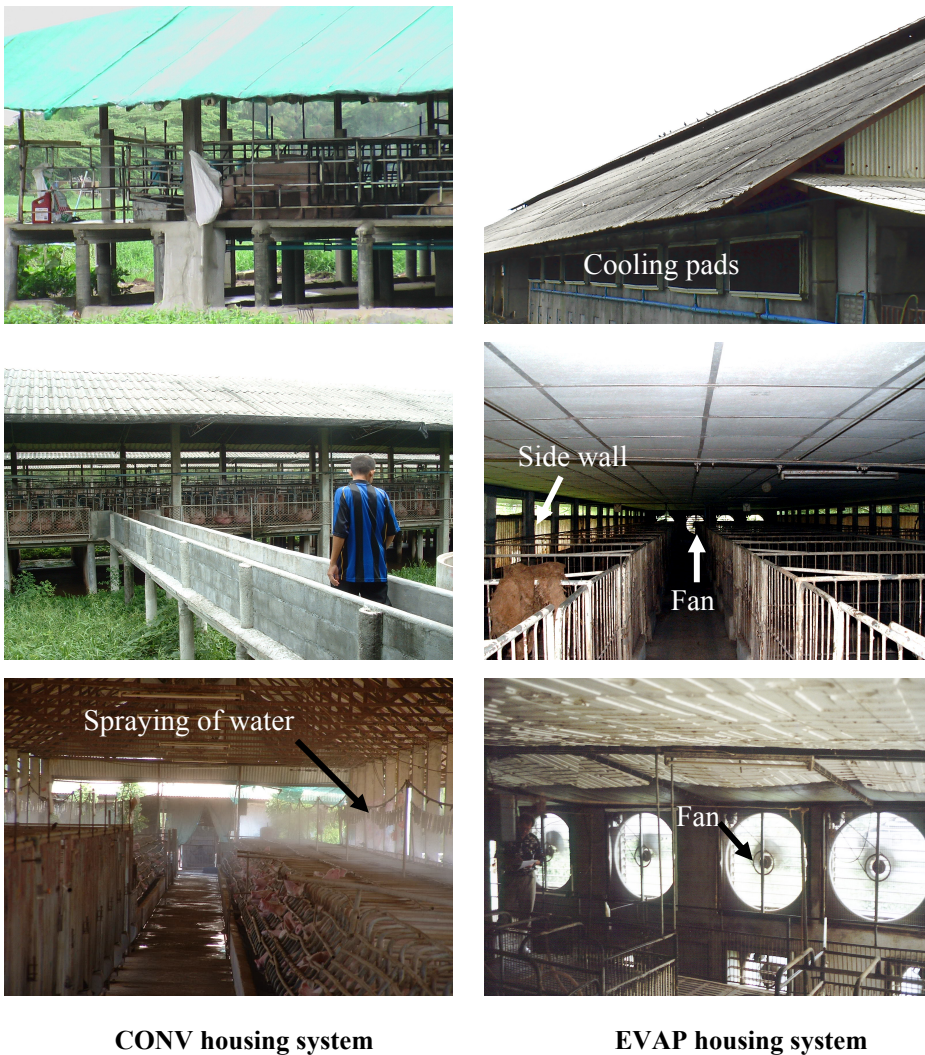
Fig. 2. Two pig housing systems: a conventional system (CONV) and an evaporative cooling system (EVAP).
