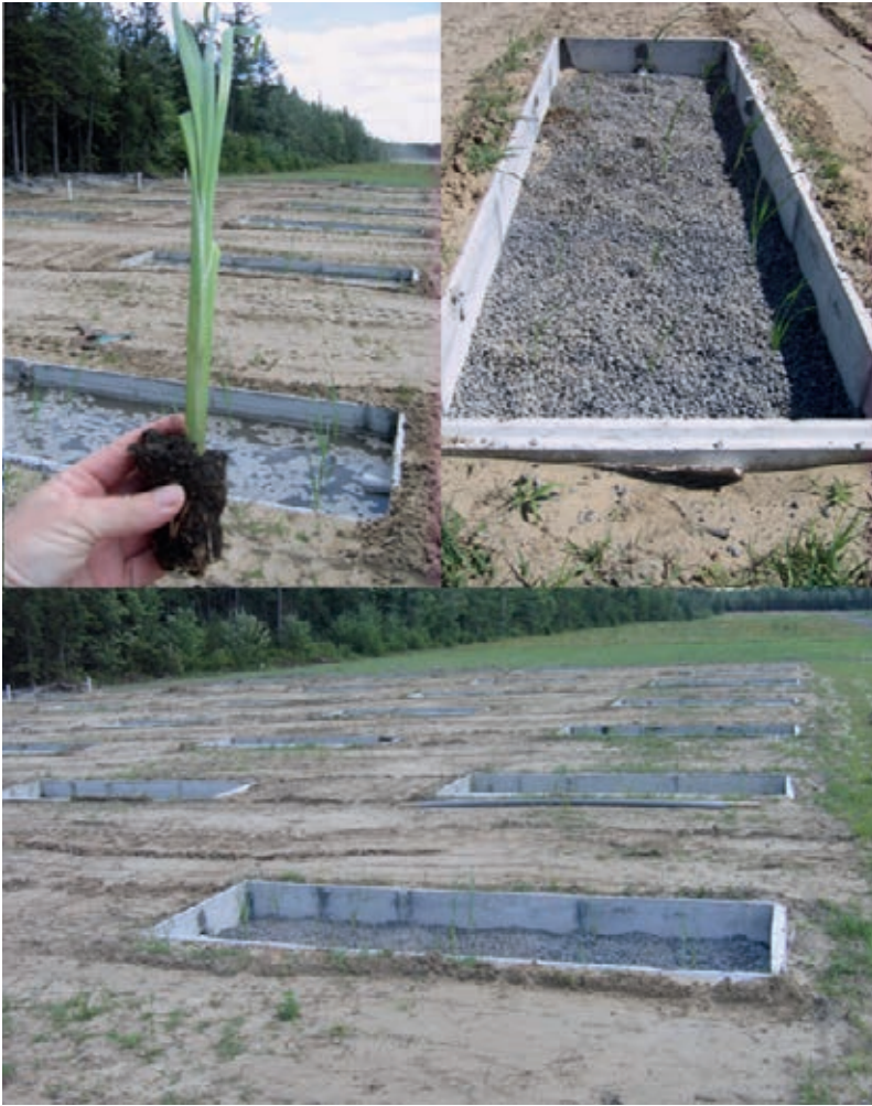
Figure 17 Horizontal subsurface flow artificial wetland units colonized with Typha latifolia to treat greenhouse effluent coming from tomato crops (photos: Martine Dorais).
