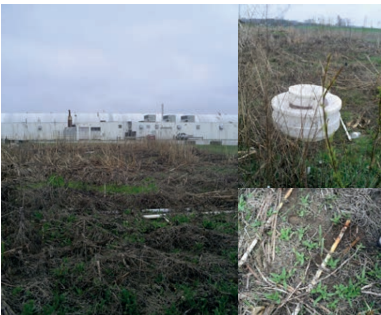
Figure 19 Vertical subsurface flow artificial wetland to treat greenhouse effluent coming from ornamental crops. (photos: Martine Dorais).
