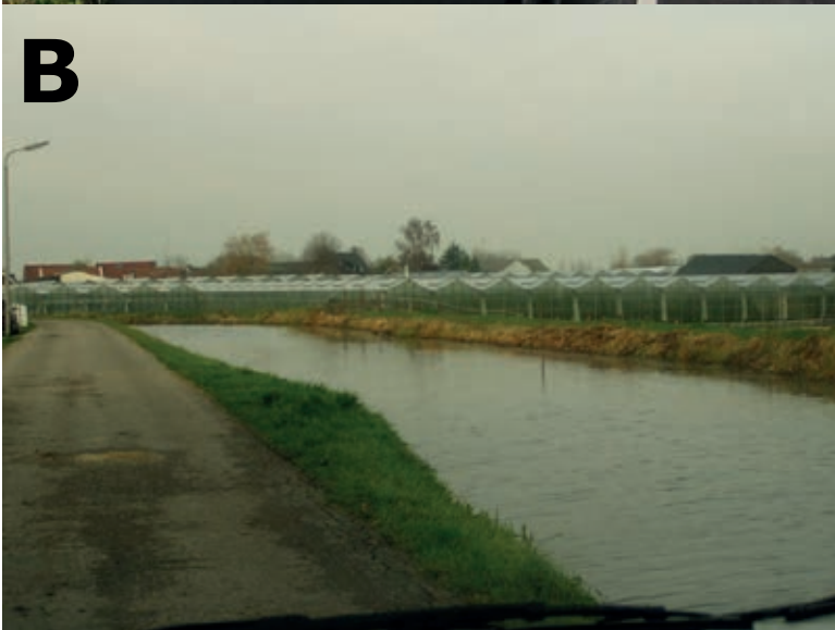
Figure 6 Rainwater management for irrigation. A: Rainwater storage as a high quality source of irrigation water; B: Potential seepage can complicate the re-use of drained water (photos: Wim Voogt).
