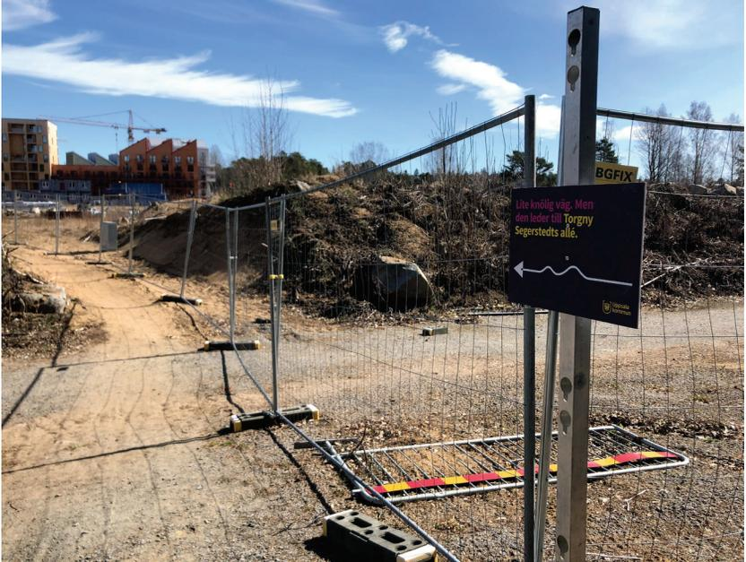
Figure 2. Fences and signs guiding pedestrians and cyclists. Photo: Bäckman, M. 2020.
