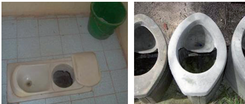
Figure 2. Dry urine-diverting toilets, Left: Squatting type made of plastic; Right: Pedestal type made of concrete, Uganda. Photos: C. Niwagaba.
