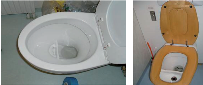
Figure 1. Double flush urine diverting toilets of different designs, Sweden. Photos: C. Niwagaba.
